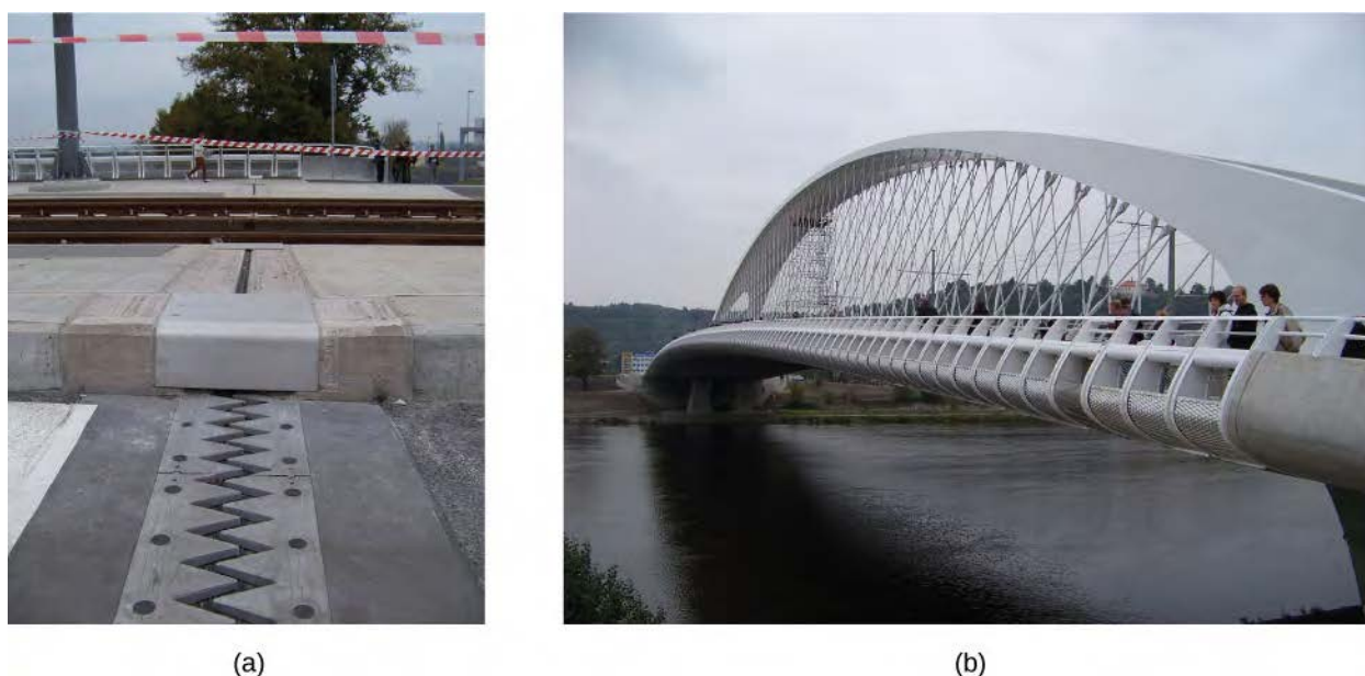
Figure 1.5 (a) Thermal expansion joints like these in the (b) Auckland Harbour Bridge in New Zealand allow bridges to change length without buckling. (credit: “ŠJû”/Wikimedia Commons)
